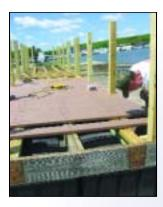
M.K. GODDARD STATE PARK The Friends of Goddard State Park provided matching funds to a grant from DCNR/PPFF to help the park replace this handicap accessible fishing pier. Park staff constructed the pier using composite decking and railing, made from 50% recycled plastic and wood, which requires less maintenance.
