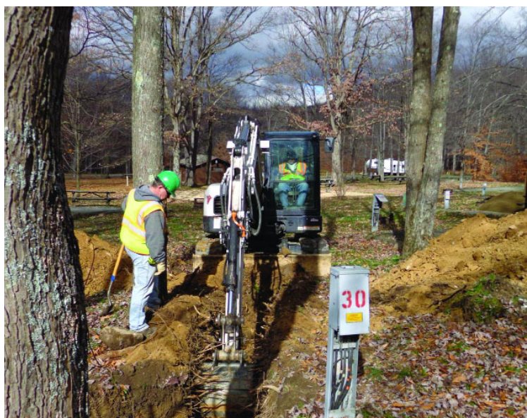
Preparing trenches for new hookups.
