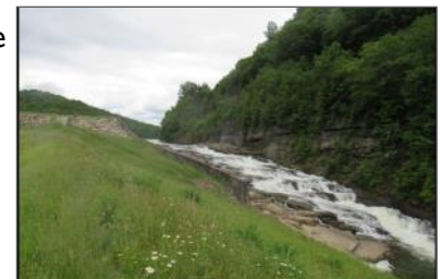
The spillway at Yellow Creek State Park's dam
