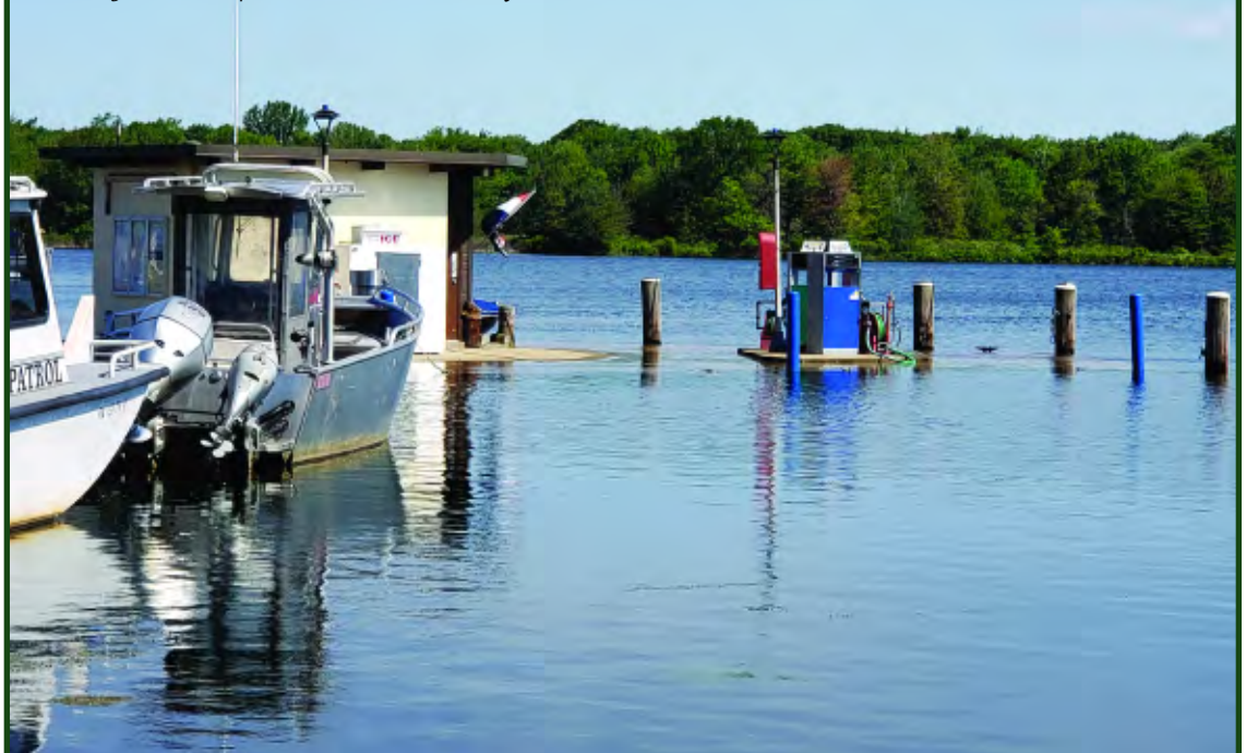
Flooding at the Presque Isle Marina due to heavy lake levels.
