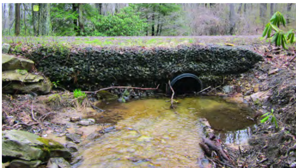
These two photos illustrate climate change adaptation. The traditional culvert design (above) is small and susceptible to washout during very heavy rain events. The new design (below) withstands heavier flooding events and is also bottomless, thereby allowing the movement of aquatic species up and down the stream.
