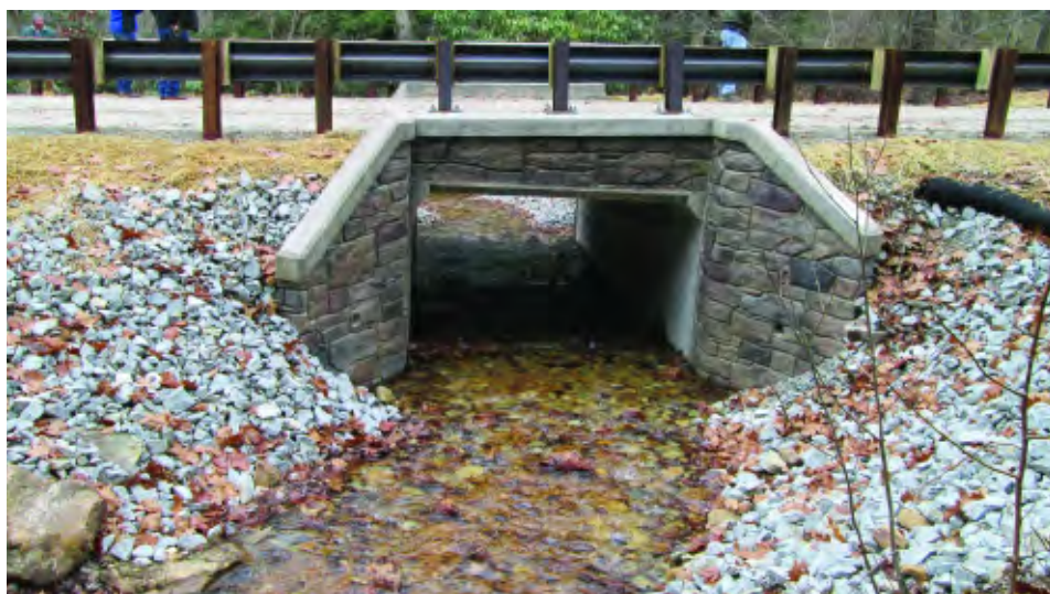
These two photos illustrate climate change adaptation. The traditional culvert design (above) is small and susceptible to washout during very heavy rain events. The new design (below) withstands heavier flooding events and is also bottomless, thereby allowing the movement of aquatic species up and down the stream.
