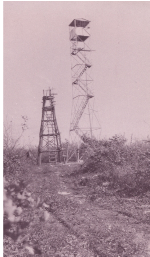
An old wooden tower is replaced by a new steel tower. Date and location unknown.
