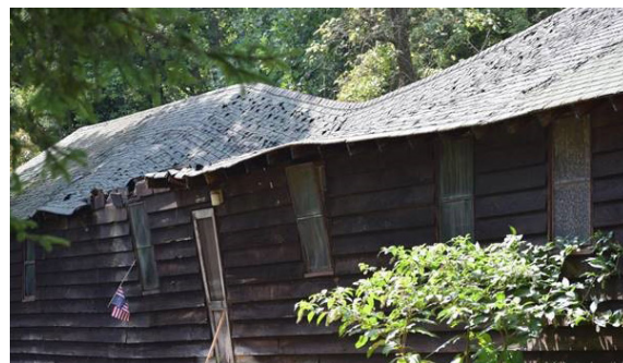
The roof of the CCC cabin collapsed unexpectedly while funds were being raised for the building preservation. Photo by DCNR
