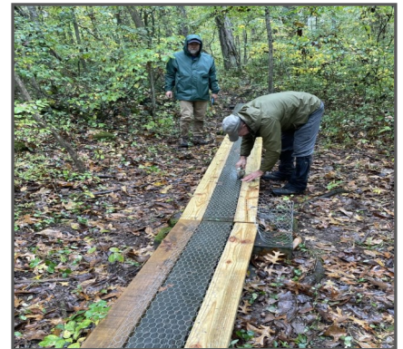
Adding chicken wire to boardwalks for increased grip and safety
