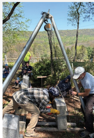
PA Outdoor Corps member, Joselyn Pena, learns to use a tripod to safely lift and maneuver heavy gravestones.
