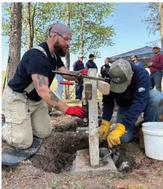
PA Outdoor Corps Leader, Quinn Ritter, and member, Jack Ridenour, mortar a fallen headstone back into the appropriate base.
